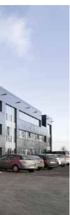
The B+T headquarters in Rechtenbach with central administration offices and adjoining factory.
