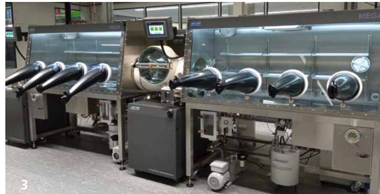
Safe cell manufacturing with glove boxes at ZESS-Technical center.
