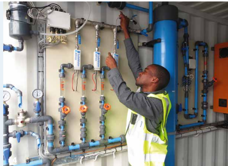
Electrode assembly of the SafeWaterAfrica system in Ressano Garcia, Mozambique
